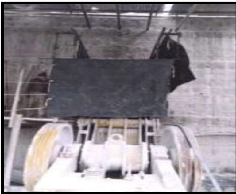
Figure-1: Covering of Primary/Jaw crusher
